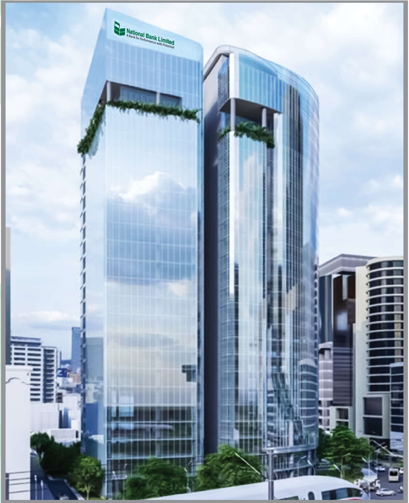
NBL Twin Tower (Under Construction) at Kawran Bazar
